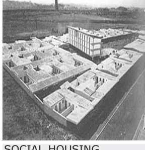
SOCIAL HOUSING VARIOUS ARCHITECTS
